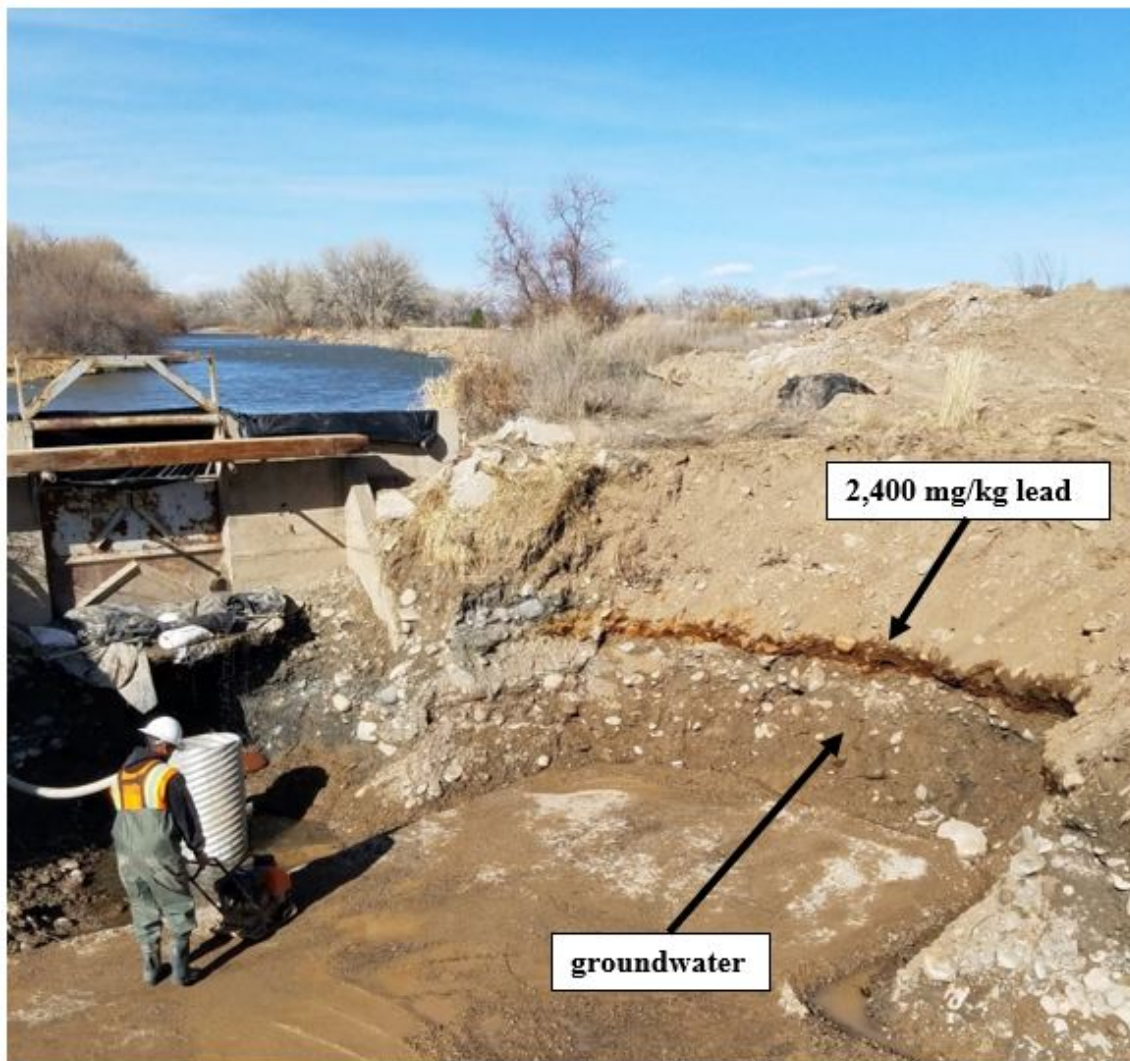
Figure 6. Lead-Contaminated Mineral Layer Along the Water Table of the Alluvial Aquifer Near Aztec (March 2016).
